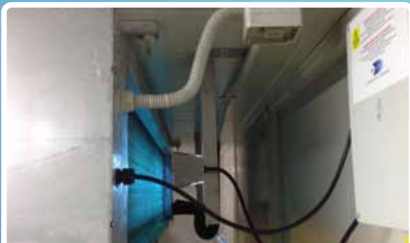
UVSNZL Evaporator Shield keeps cool room evaporator coils clear and free from microbial contamination
